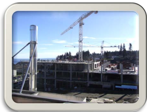
Campbell River Hospital – New Build in Progress
