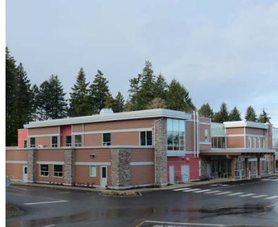
Oceanside Health Centre
