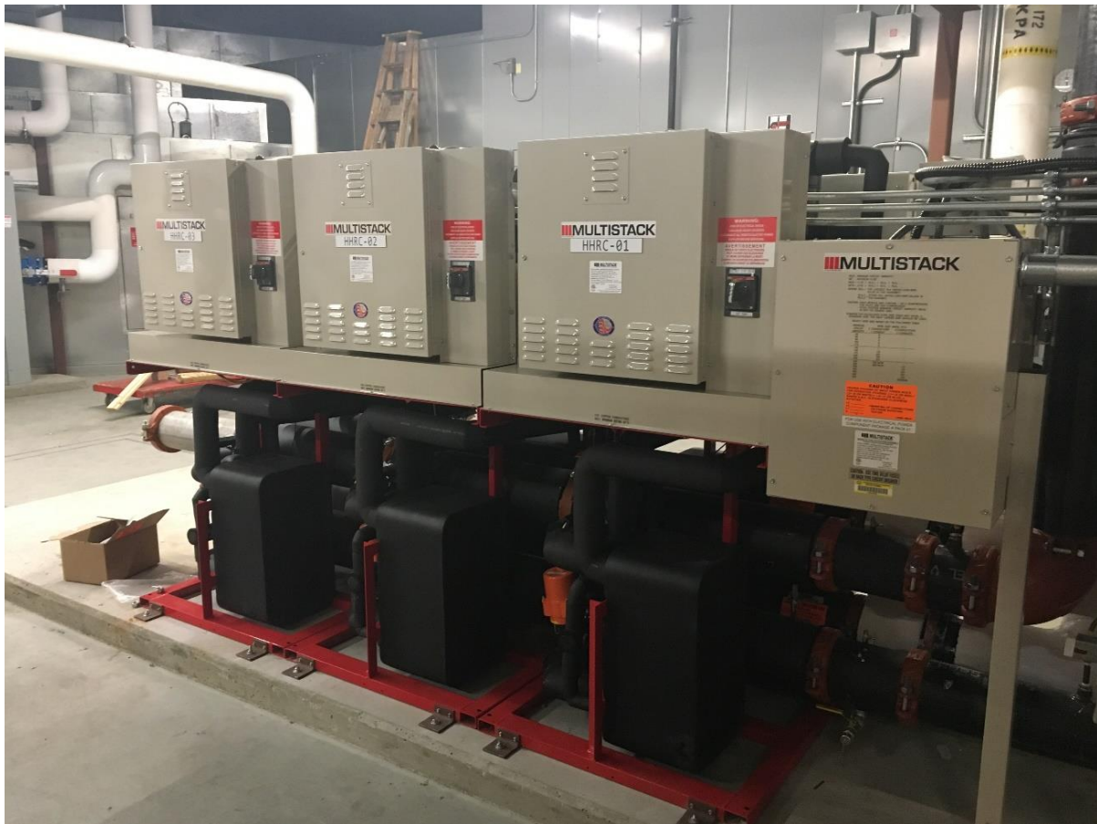
(Image of the heat recovery chiller installed during the Royal Jubilee Hospital D&T Heat Recovery Chiller Phase 1 project.)
